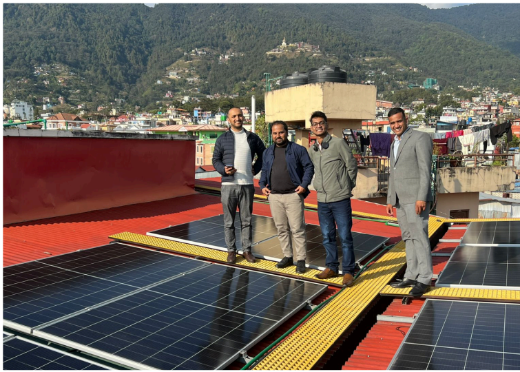
Truvalu team visit to Park Village, Kathmandu - A Gham Urja solar installation
